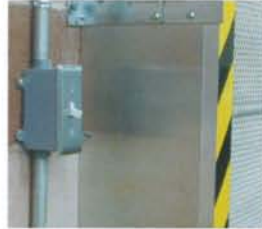
Metal sheeting covers the side of the guide tracks to provide a secure seal.
